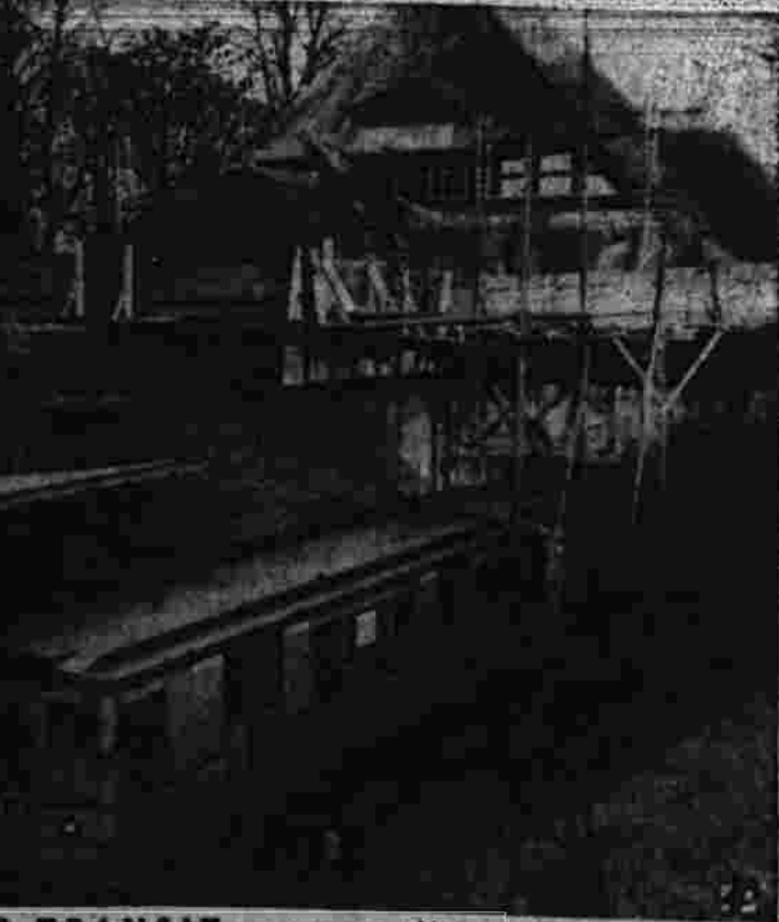
BEAUTIFYING RAPID TRANSIT —Workers build what may appear to be a rural farmer's home but is really the gateway station in the Babylon district of West Berlin.
